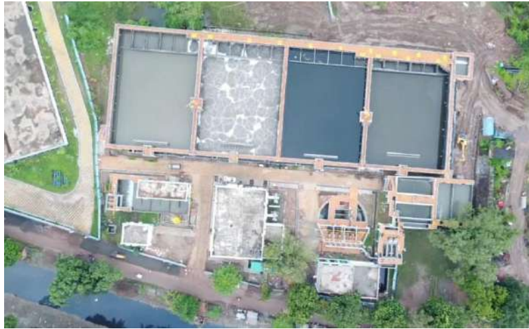
35.00 MLD STP at Maheshthala, Kolkata
