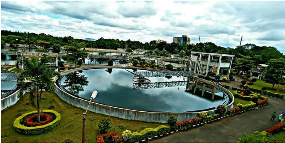
115.00 MLD STP at Naidu, Pune
