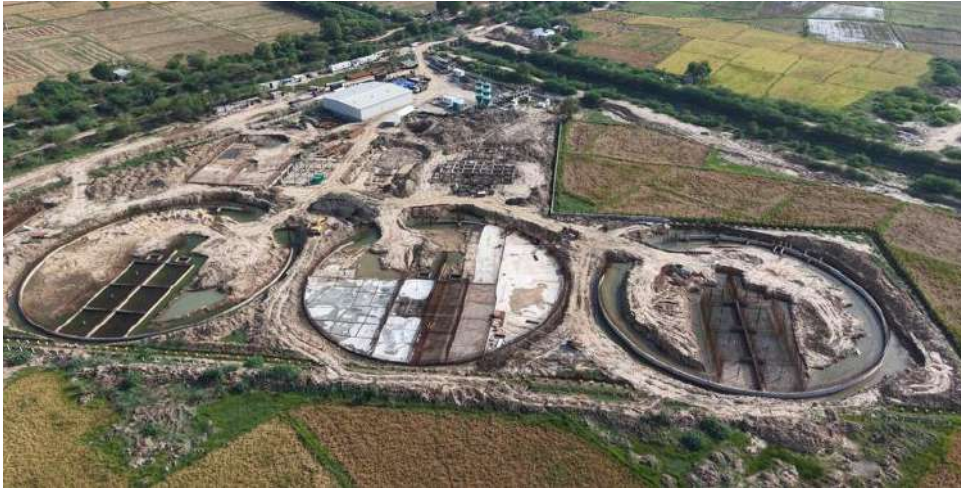
107.00 MLD STP at Ahmedabad, Gujarat
