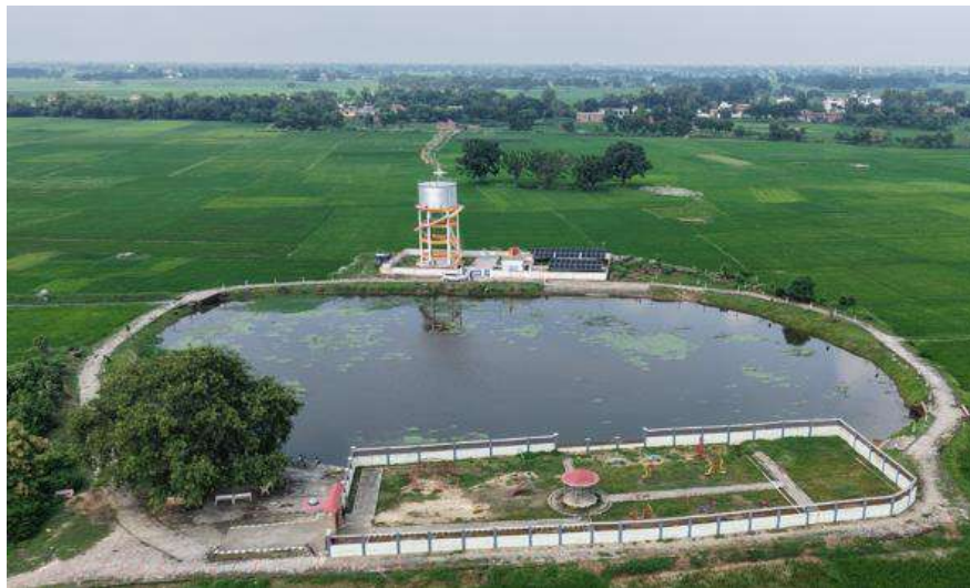
Water Supply Scheme at Sant Kabir Nagar
