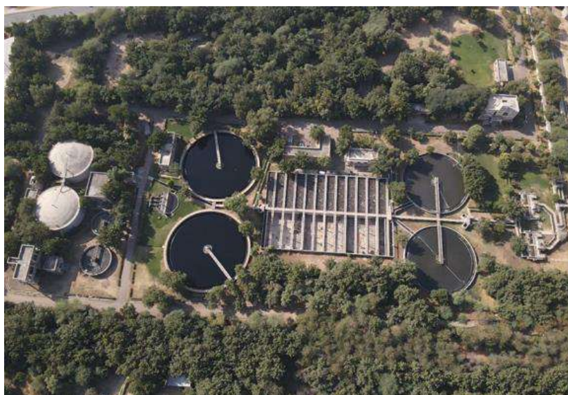
50.00 MLD STP at Salawas, Jodhpur
