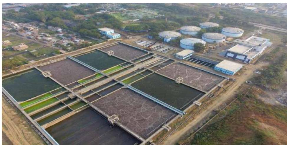
Bhandewadi 200.00 MLD STP and 190.00 MLD Reuse Project (Phase I and II)
