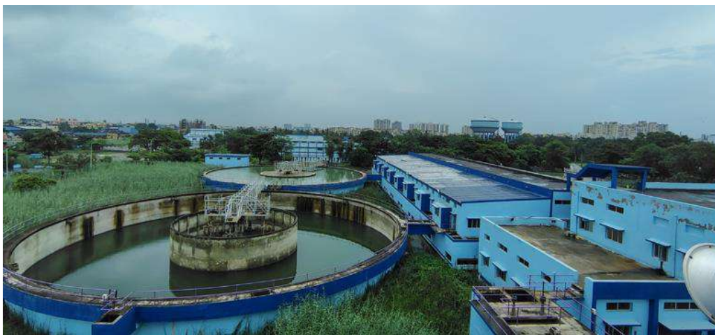
113.50 MLD WTP at Baranagar, Kolkata
